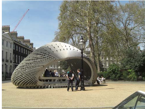
Fiber reinforced concrete (approx. 2% vol.) : 500 time more resistant to cracking and 40 % lighter in weight
