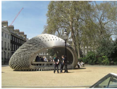
Fiber reinforced concrete (approx. 2% vol.) : 500 time more resistant to cracking and 40 % lighter in weight
